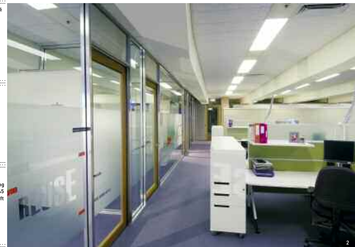
1_View of hard wood entry feature wall (built by Schiavello) through to waiting area, and glazed Millem partition system. 2_Millem finished aluminium glazed partition system with feature window film and full glass cedar doors leading into workstation area including QED desking and tambour units using MDF powder coat technology. System 45 feature with their translucent panels and soft curved power rails.
