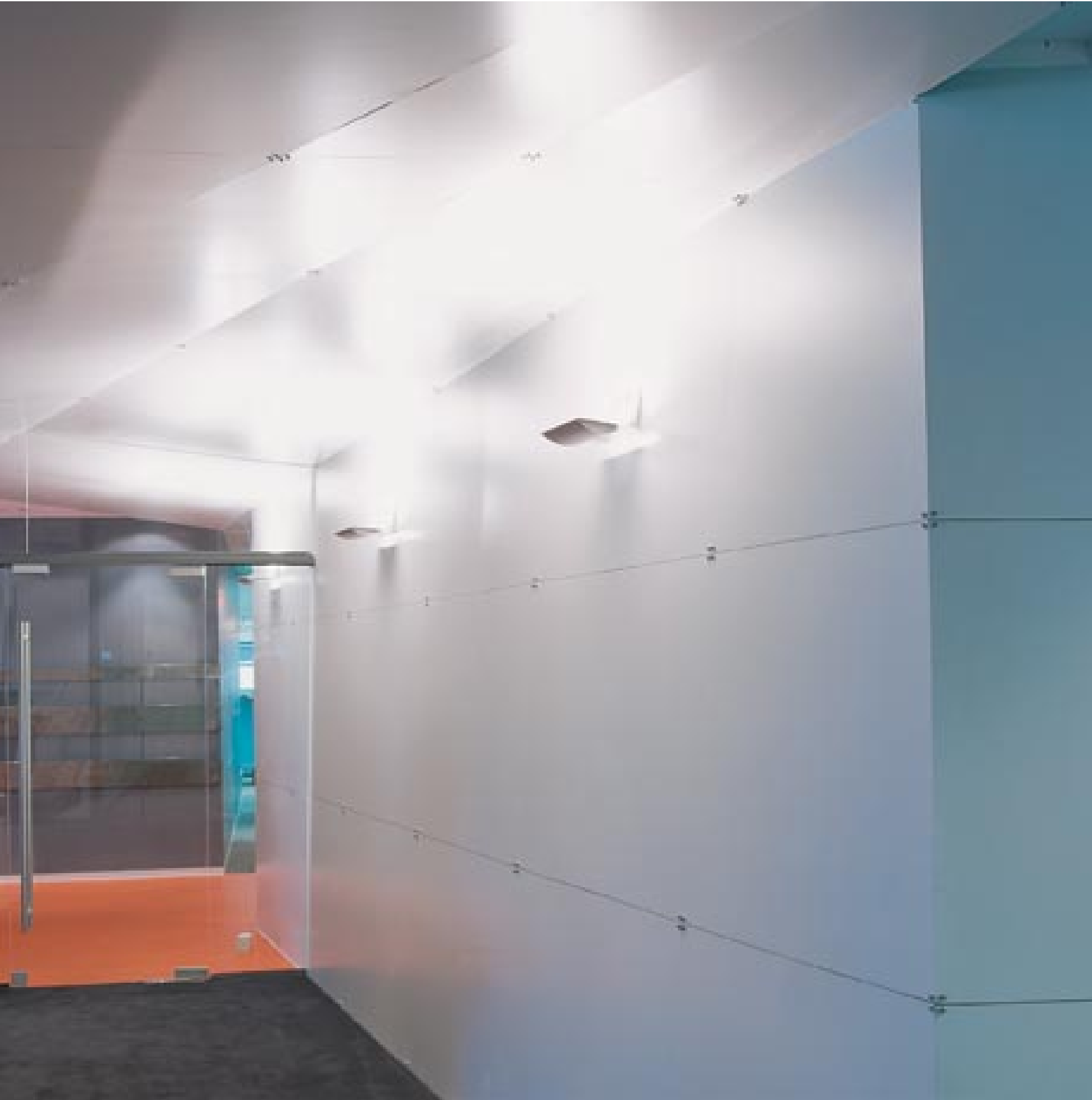
Above ... Reception ceiling + angled walls in BHP steel Colorbond sheet.
