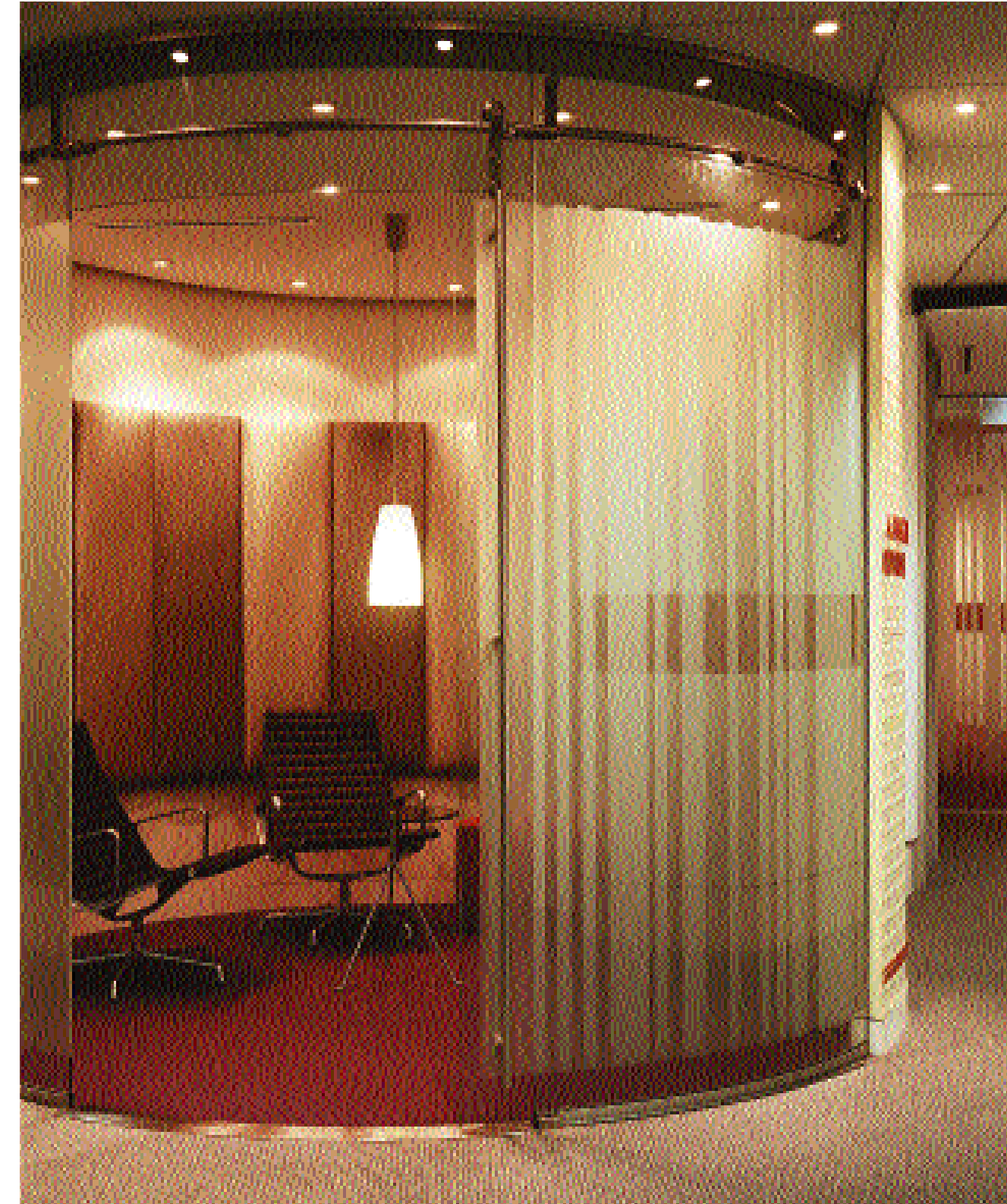
Above Image Frameless glazed curved sliding doors and detailed curved joinery.
